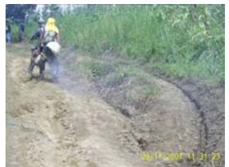
Severely damaged road
