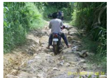
Road very dangerous to maneuver
