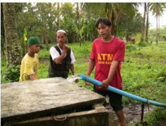
The intake box at Brgy. Piangologan having the same source of water spring
