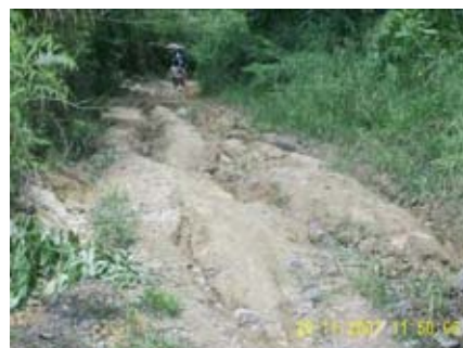
Line canal should be constructed at both sides of road to protect water run-off from running on different directions
