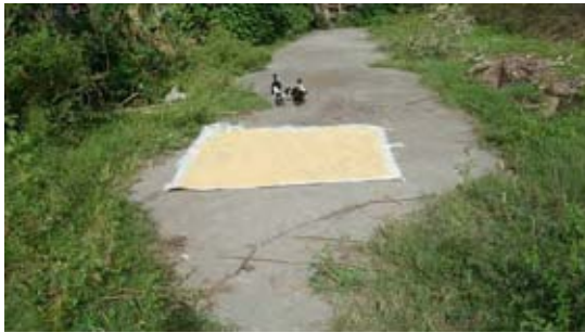
Farmers are using the concrete pavement as dryer of their produce
