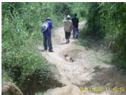
Road side needs to be slope protected
