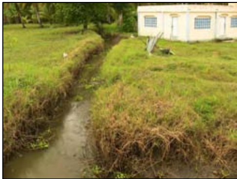
Construction of lined canal along this creek
