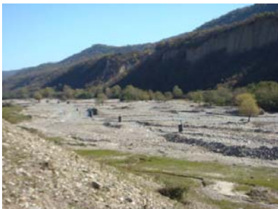
1. Intake facility at Old 18km site
