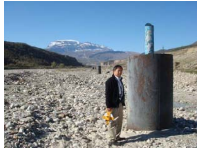
2. Connecting chamber of New 18km site
