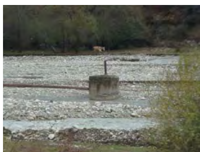
4. Connecting chamber of 7km site
