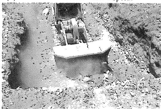
(3) Apply cover soil onto the waste
