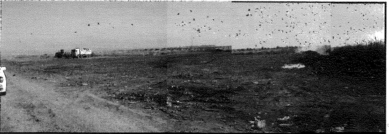
January 22 and 23, 2007: After removal of the existing waste to the wadi side
