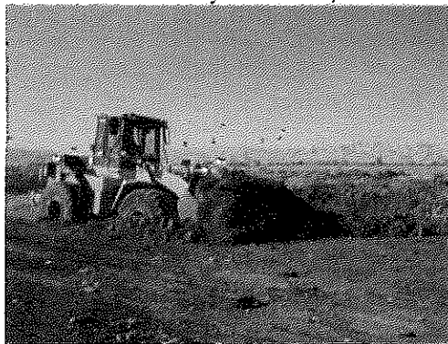
January 24, 2007: Start of excavation works
