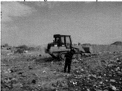
Mr. Roma, Head of technical section, instructs and supervises landfill works.
