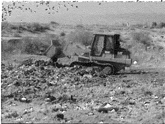
Spreading of waste and compaction
