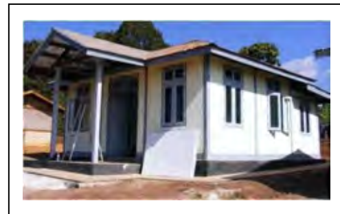
Maw Mar Sub-RHC after renovation
