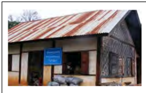
Maw Mar Sub-RHC before renovation
