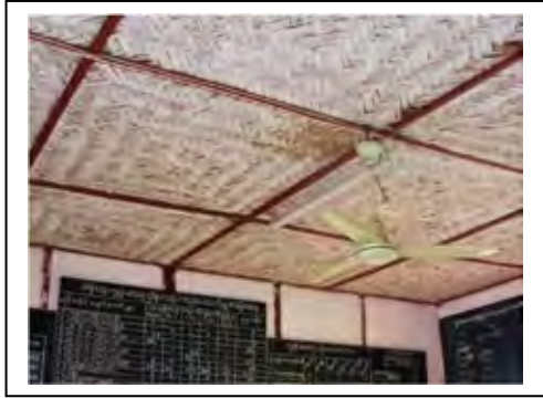
Bant Bwe RHC before renovation
