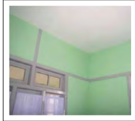
Bant Bwe RHC after renovation
