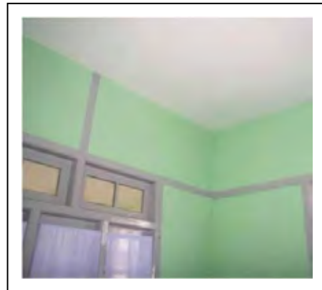
施設改修後(Bant Bwe RHC)
