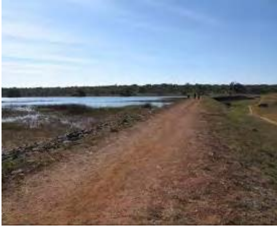
Figure D.22 Existing Lusiwasi dam
