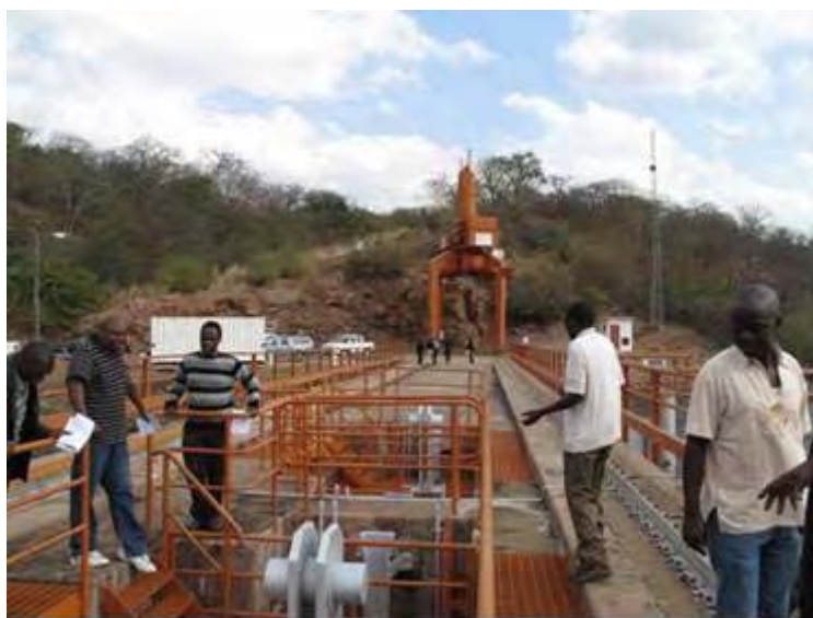
Figure D.3 Gates of diversion tunnels (Future intake gate)
