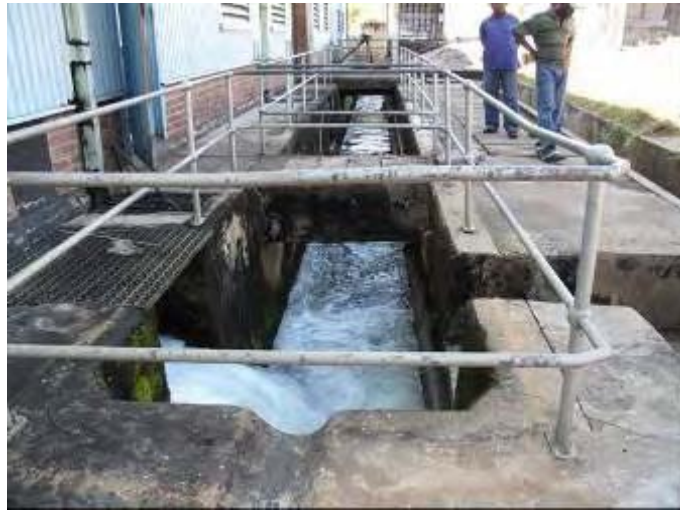
Figure D.19 Existing tailrace
