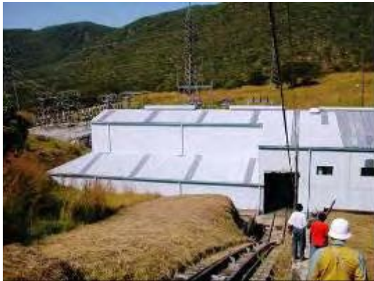
Figure D.17 Existing power house
