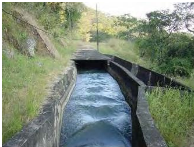
Figure D.14 Existing headrace
