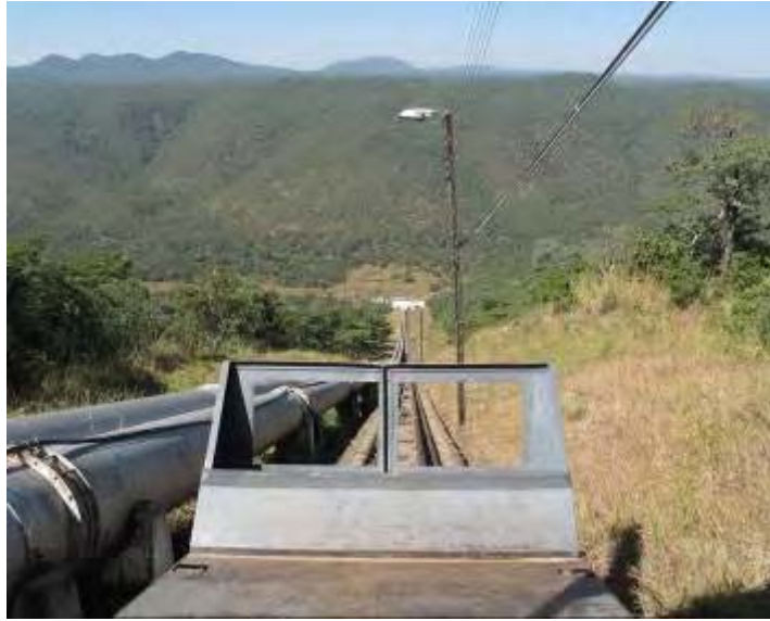
Figure D.16 Existing penstock
