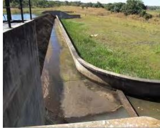
Figure D.23 Overflow part of the existing Lusiwasi dam
