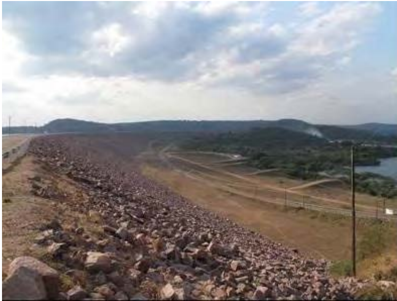
Figure D.1 Itezhi-Tezhi dam downstream face (view from the right edge)
