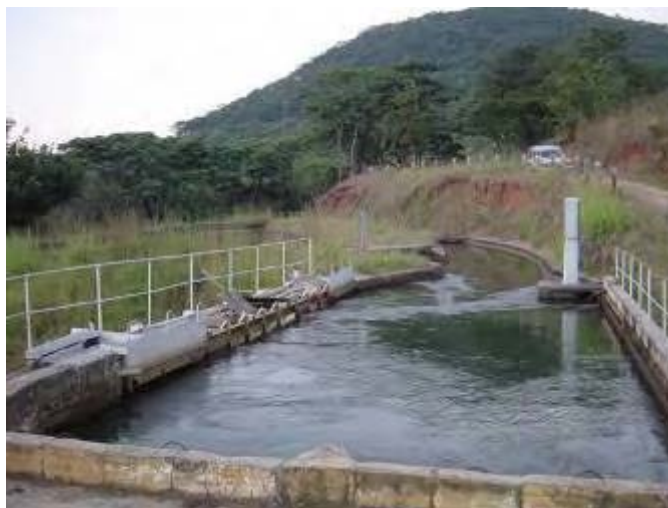
Figure D.15 Existing head pond
