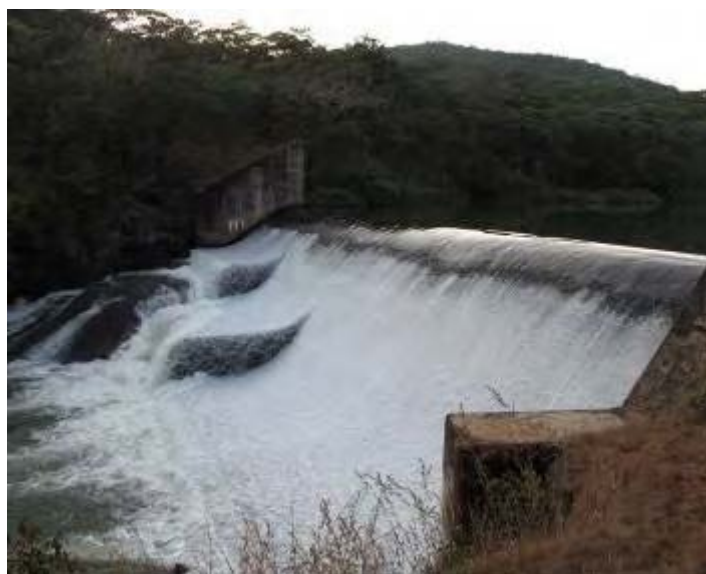
Figure D.13 Existing weir
