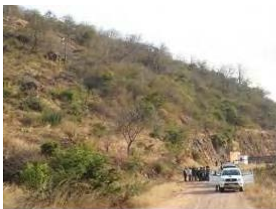
Figure D.4 Power station construction site
