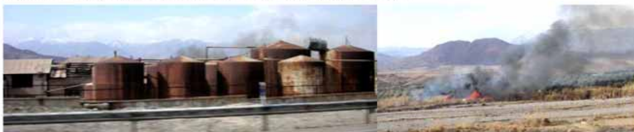
Photo-10: Cause of Water Quality Deterioration
