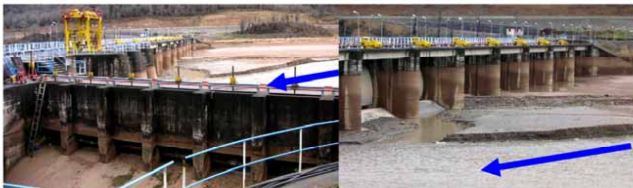
Photo-17: Upstream Condition of Tarik Diversion Dam
