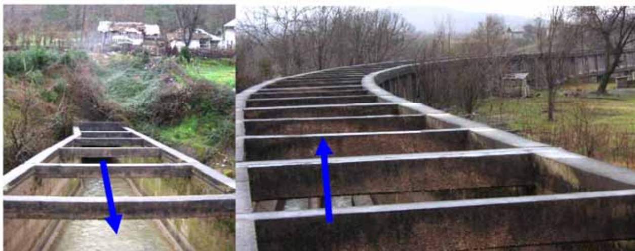
Photo-20: Outlet of Intake Tunnel and Adjacent Main Canal
