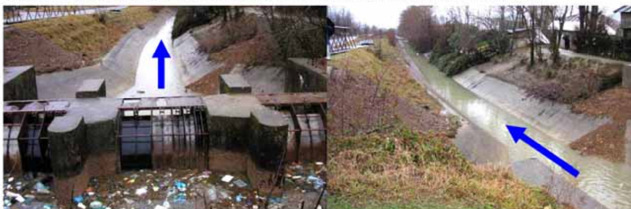
Photo-23: Intake Gate of Secondary Canal and Secondary Canal
