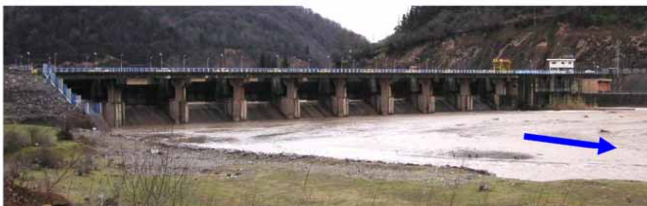
Photo-17: Tarik Diversion Dam on the Sefidrud River
