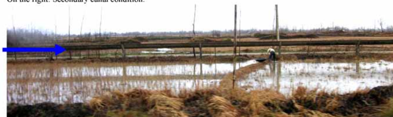
Photo-24: Flume-type Tertiary Canal and a Farmer in the Paddy Field for Preparation of Cultivation
