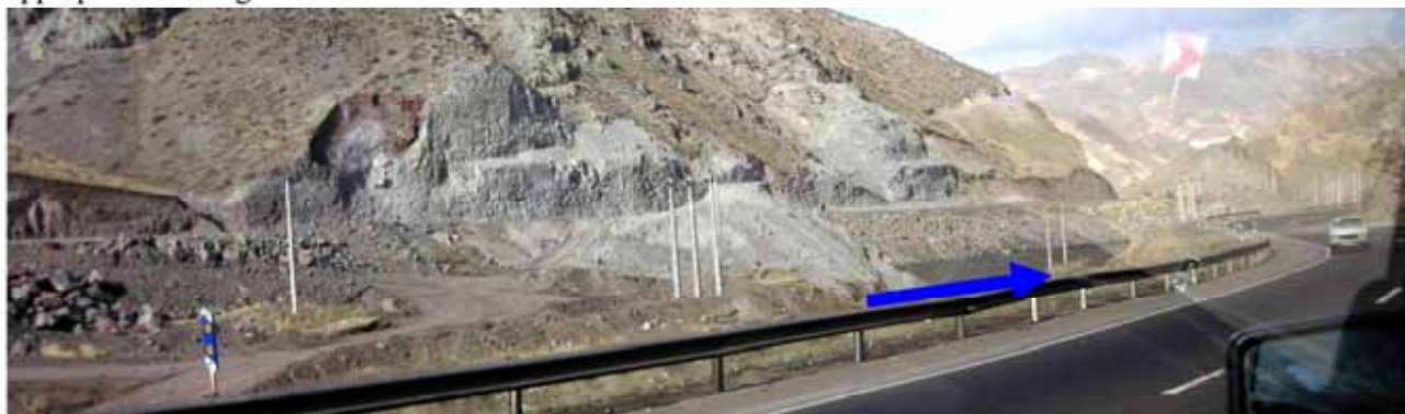
Photo-5: Creation of New Sediment Deposit by Road Construction
