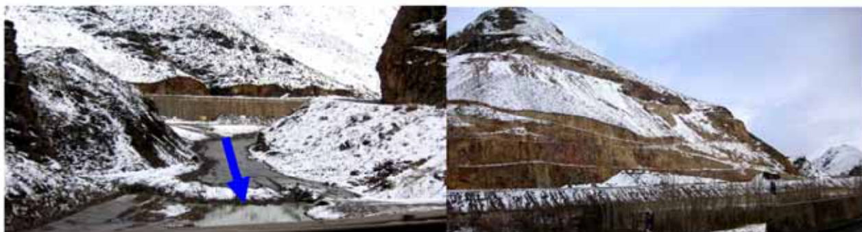
Photo-6: Creation of Sediment Deposit by Road Construction - 2
