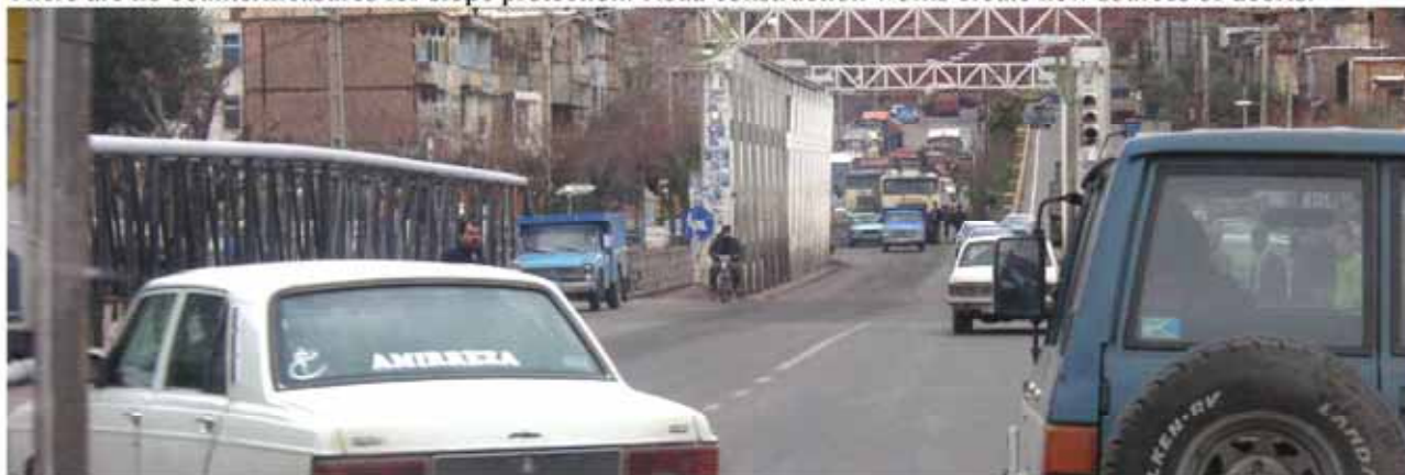
Photo-8: Bridge crossing Shahrud River at Lowshan
