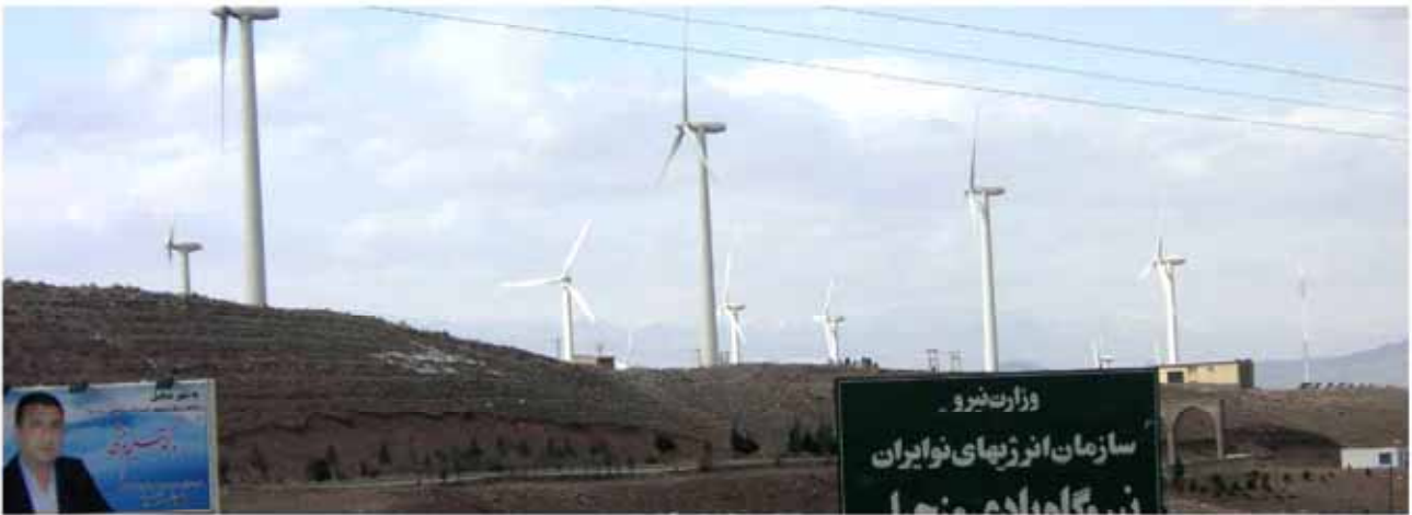
Photo-11: Wind Power on the Left Bank of the Damsite
