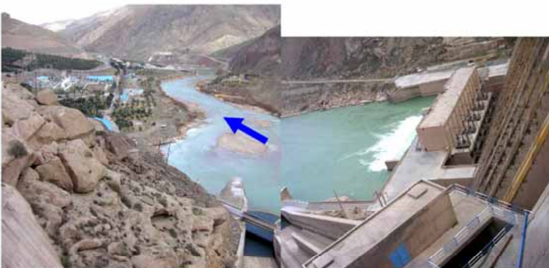
Photo-13: Downstream view of Manjil Dam-2
