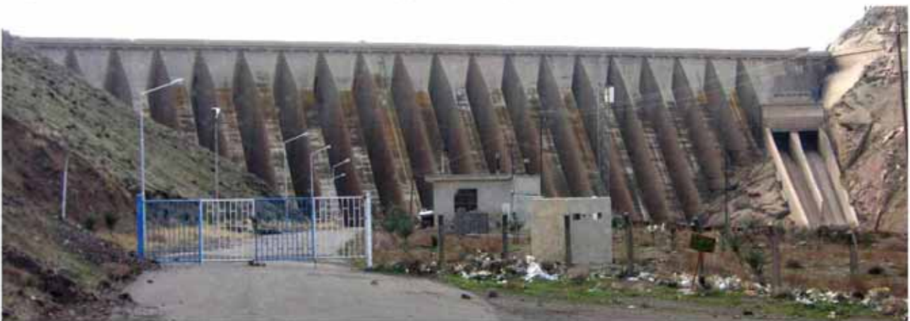
Photo-12: Downstream view of Manjil Dam-1
