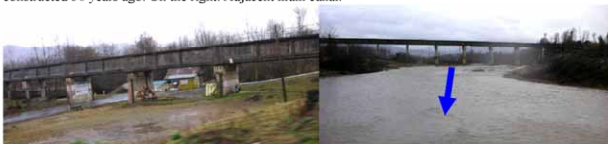
Photo-21: Aqueduct Bridges of the Main Canal
