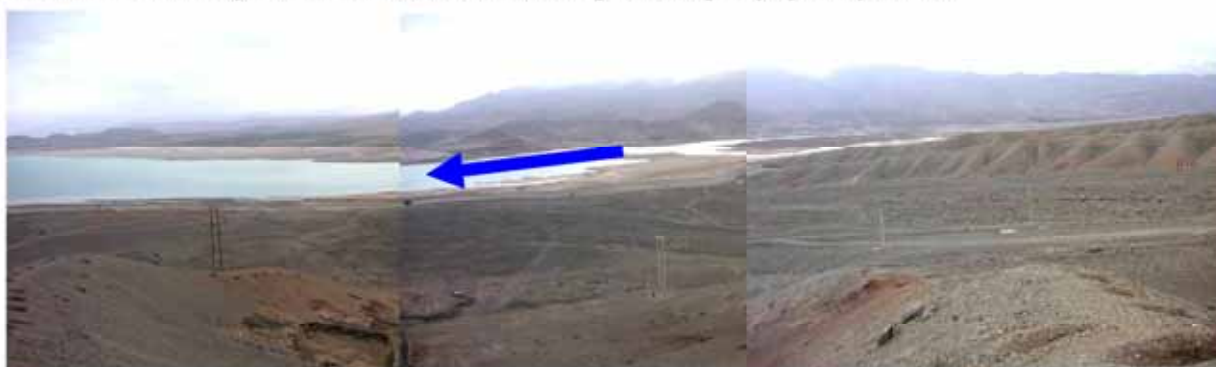
Photo-15: Sedimentation of the Reservoir on the Left Tributary, the Qezl Owzan River
