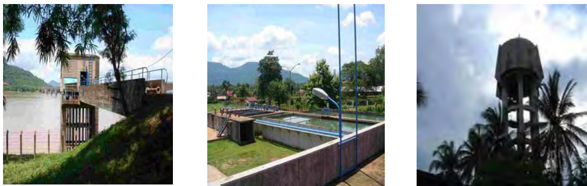
Figure 3.13 Existing Water Intake Tower, Water Treatment Plant and Elevated Water Tank
