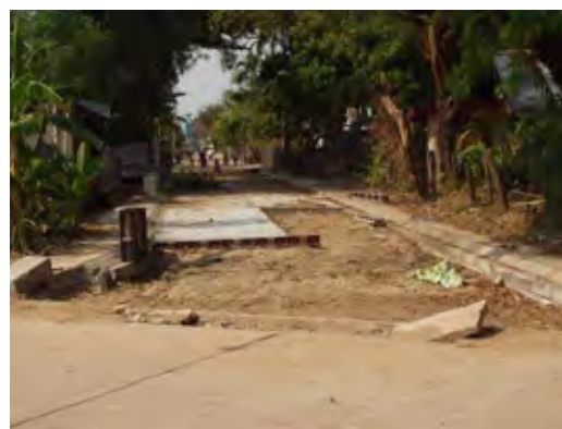
Local road under construction
