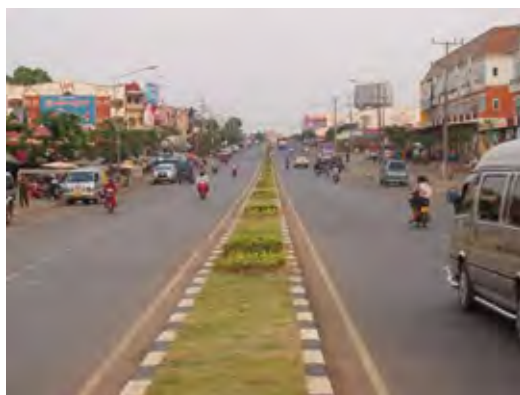
Road No38 constructed at the downtown – a southern bank of Xedong River
