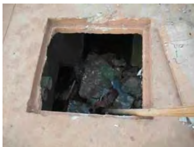
Drainage in Pakse
