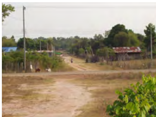
Unpaved road in urban area
