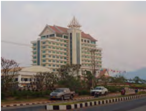
Hotel constructed at the riverside
