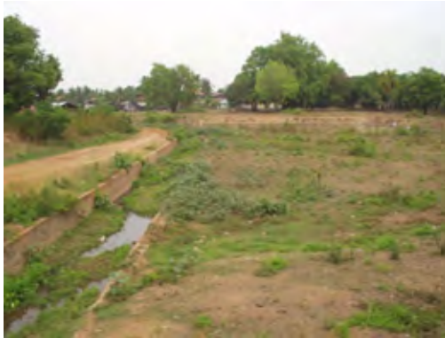
Improper development of stream bank
