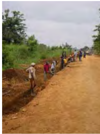
Excavation for side ditches by manpower
