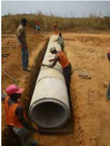
Placing of crossing culvert
