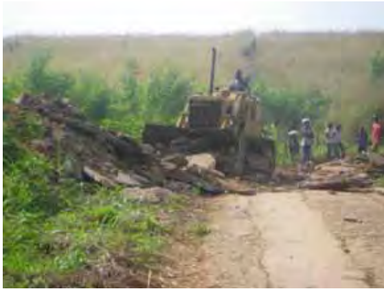
Demolition of existing concrete pavement
