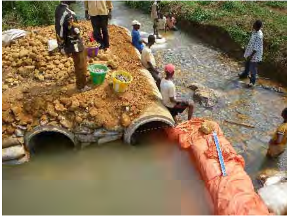
Temporary road at bridge
