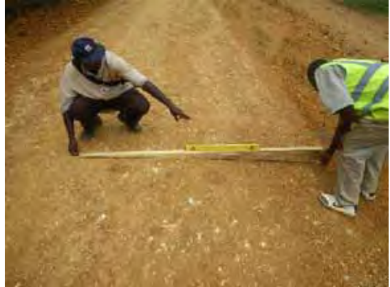
Check of transverse slope
