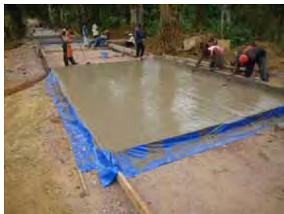
Casting and Finishing of concrete
