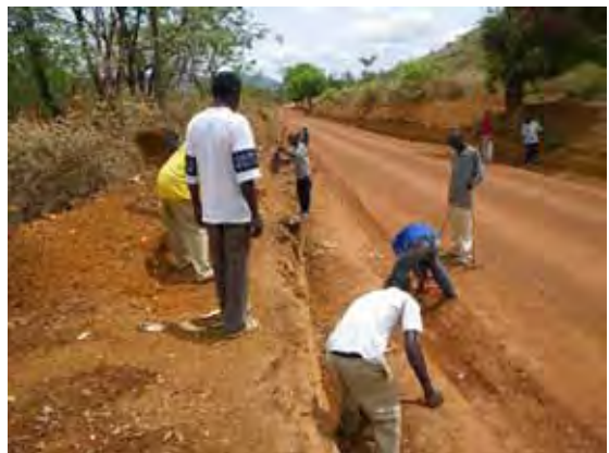
Practice of maintenance of side ditches
