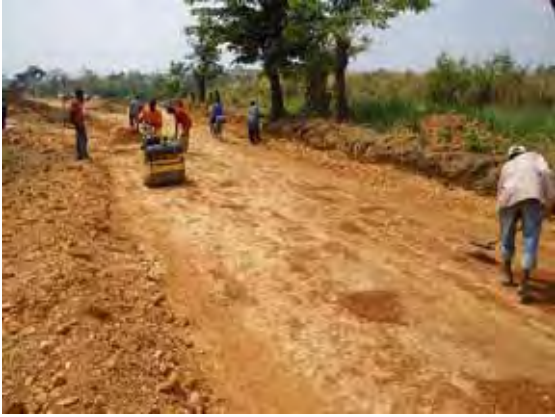
Finishing of laterite pavement
