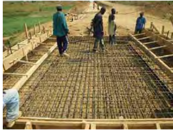
Placing of reinforcement bar (No.3 bridge)
