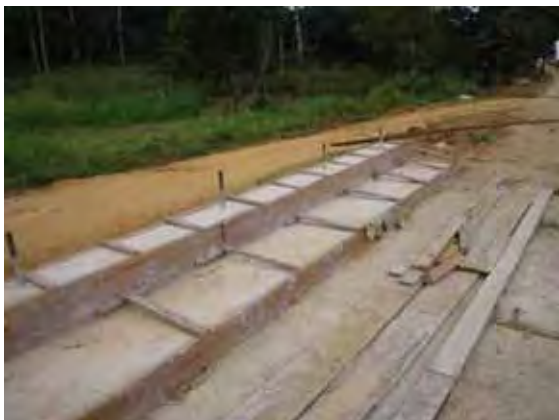
Foot path (No.1 Bridge)
