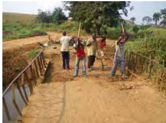
Demolition of a part of existing bridge
