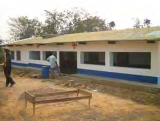
Repaired health center of Malanga Cité
