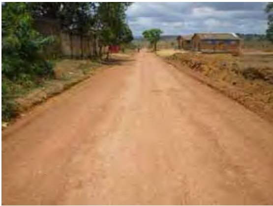
Finishing of laterite pavement
