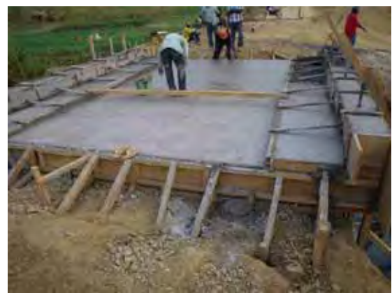
Cast of concrete (No.3 Bridge)
