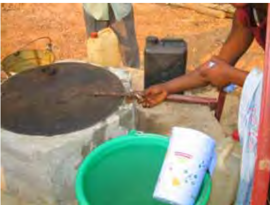
Completed well of Mawewe. A padlock was attached for the control
