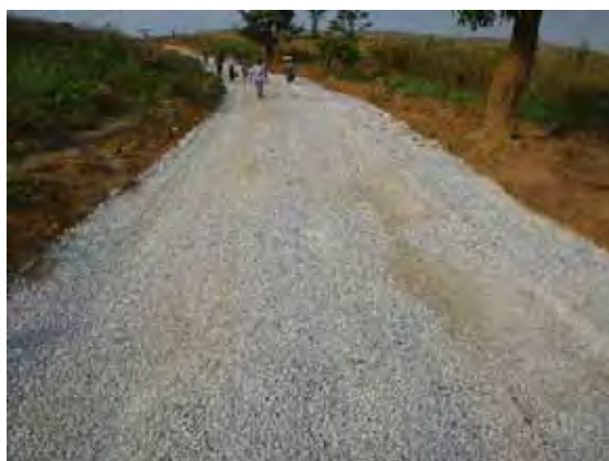
Setting of base course (using crusher run)
