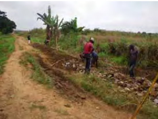
Finishing of laterite pavement (Kimpese city)
