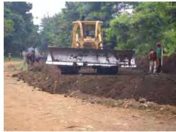
Extention of existing road
