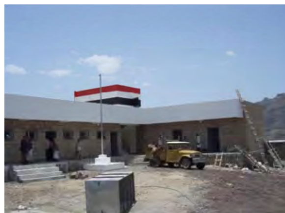
School construction in Al Marfa
