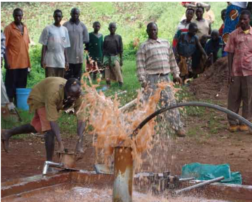
Local residents watch as the well interior is cleaned.
