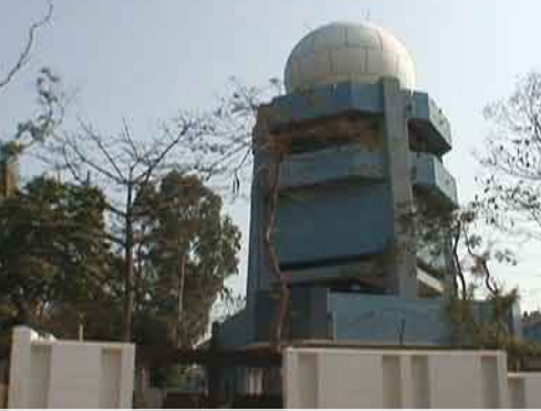
Weather radar installation (Bangladesh)
