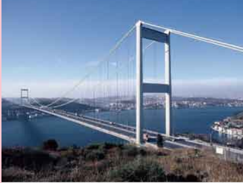
Bosphorus Bridge No. 2 (Turkey)
