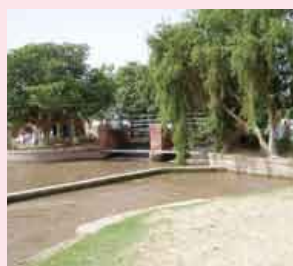
Irrigation canal in Bahawalnagar
