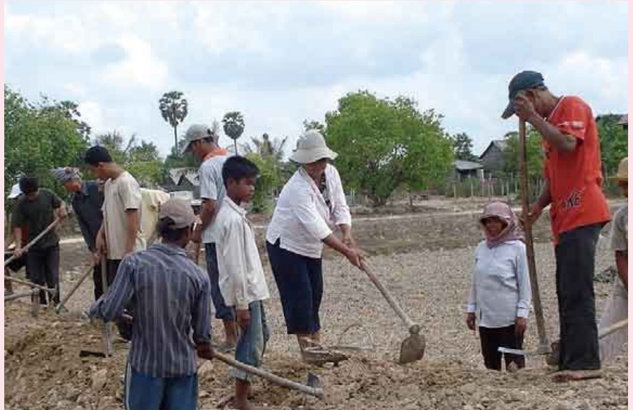
Restoring an irrigation ditch in Cambodia
