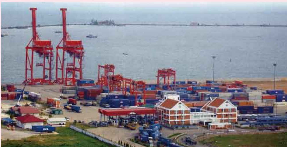
View of Sihanouville Harbor's two primary container cranes (left) and container dock (right) equipped with cooperation by JICA
