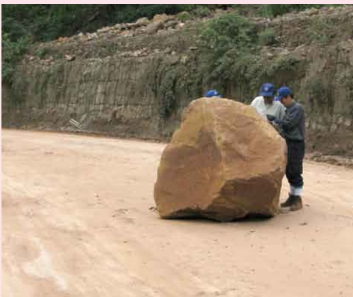
Surveying fallen boulders (size, configuration of the fall, damages)
