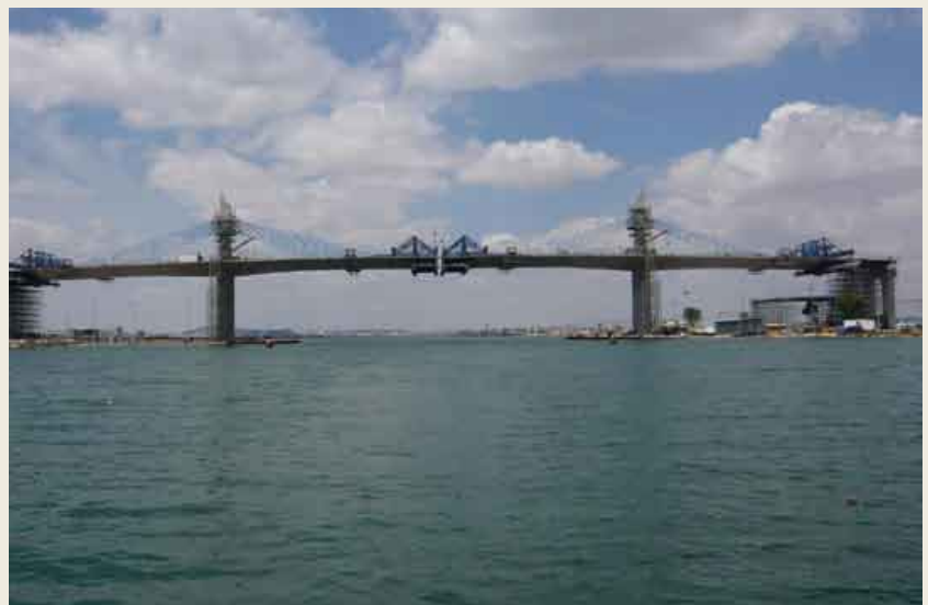
The Rades-La Goulette Bridge
