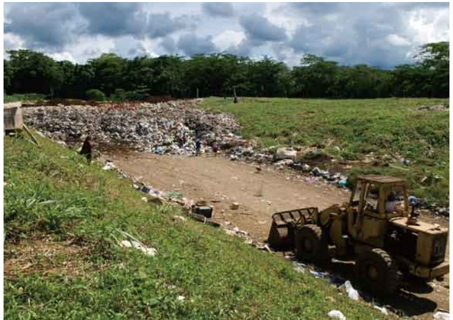
Improvement seen in Tafaigata landfill treatment facilities in Samoa after adopting the Fukuoka method. After a garbage truck arrives, scavengers pick up valuables from the collection before the machinery sweeps the garbage away for crushing and compacting.
