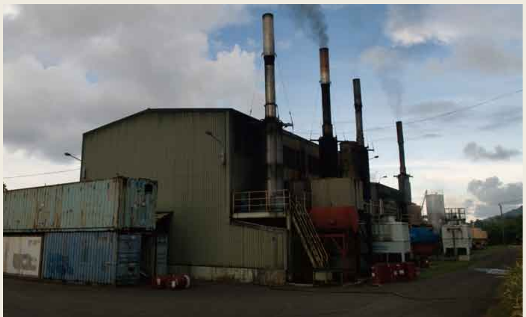
An aging thermal power plant in Apia, Samoa where new construction is scheduled thanks to JICA ODA loans
