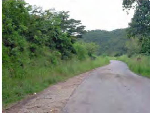
Photo 2-2-3 Condition of an Existing Cut Slope Surface
