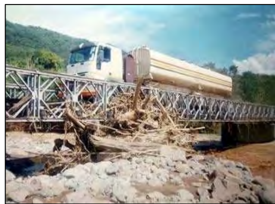
Photo 2-2-2 The Existing Rukuru Bridge Damaged by Flood
