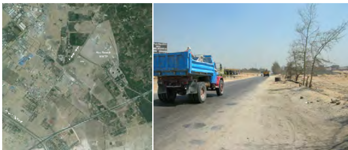
Figure 6-2 Access Road from Desert Highway to Abu Rawash WWTP
