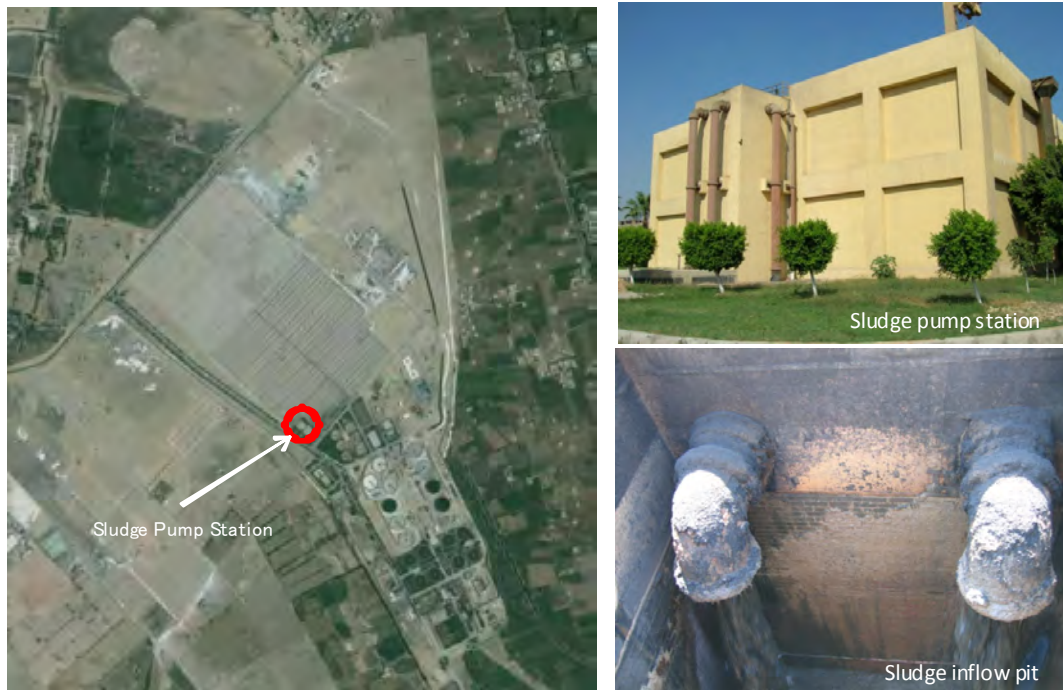
Figure 4-12 Sampling Point of Odor Measurement Survey at Sludge Pump Station
