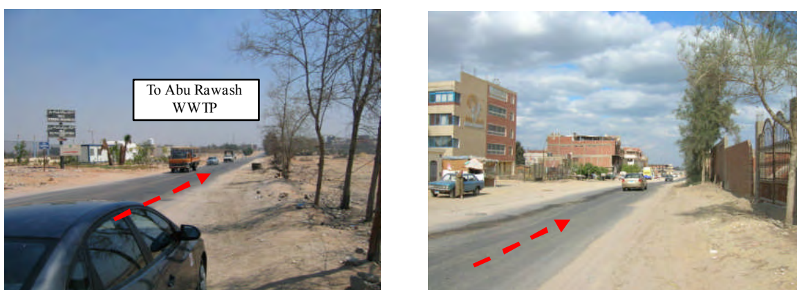
Figure 4-18 Access Road to Abu Rawash WWTP
