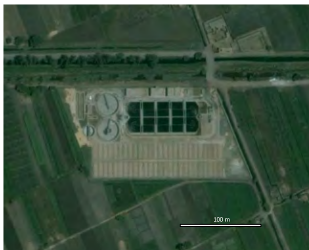
Figure 6 Outline of Manashi WWTP
