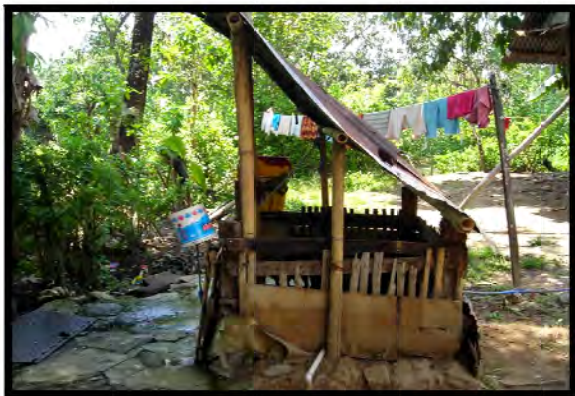
A Deep Well in Raya Village: Public Facility
