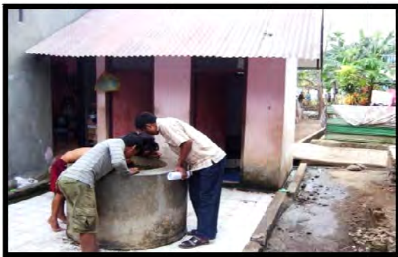
An Artesian Well & Public Toilet in Kalegowa
