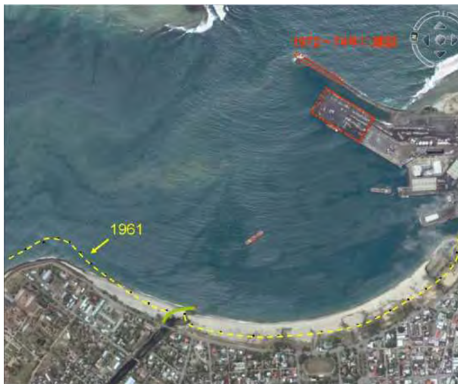
Figure 6-3-5 Superposition of the shoreline in 1961 on the recent aerial photograph
