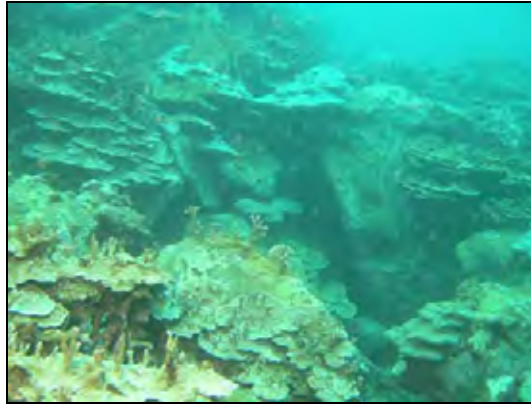
Figure 4-1-11 Coral on the Rock foundation of C3 Quay (Toamasina Port)
