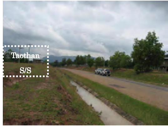
Photo-14: Route 13 Crossing Point 1
