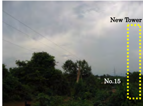
Photo-04: New T/L Crossing Point (No.14-15)
