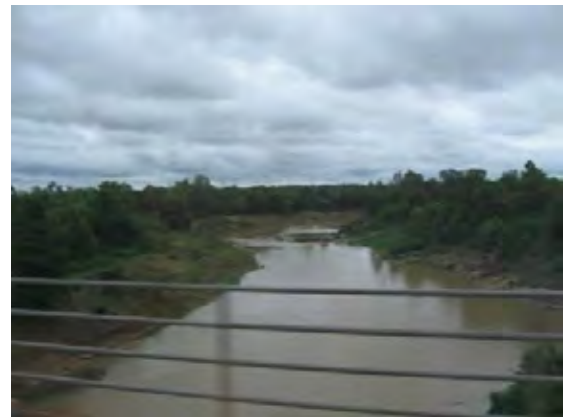
Photo-12: Xe Nouan Crossing Point 1
