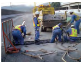
Replacement of Expansion Joint
