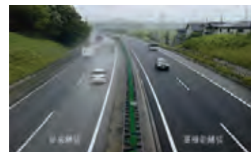
Improvement of Pavement
