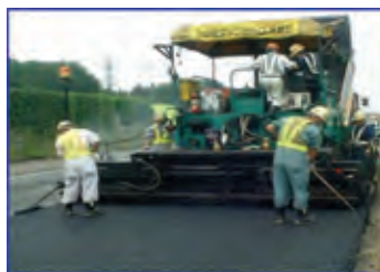
Reconstruction of Pavement
