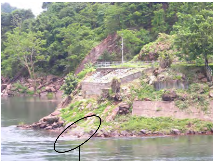
Right bank of tail bay
