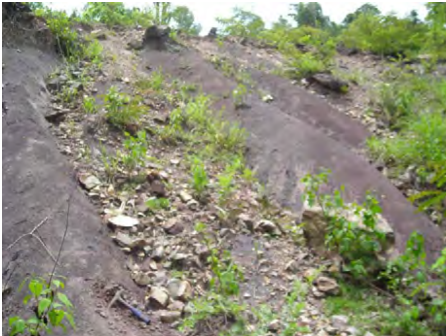
Dam site right abutment (Weak mudstone stratum)
