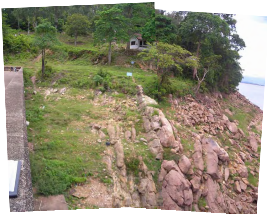
Dam site right abutment (Same stratum of the dam foundation sandstone)
