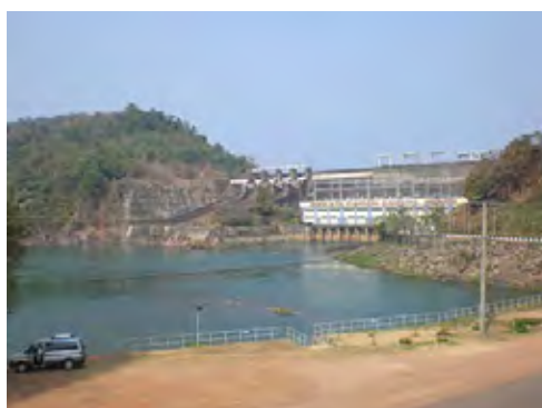
NN1 Hydropower Station
