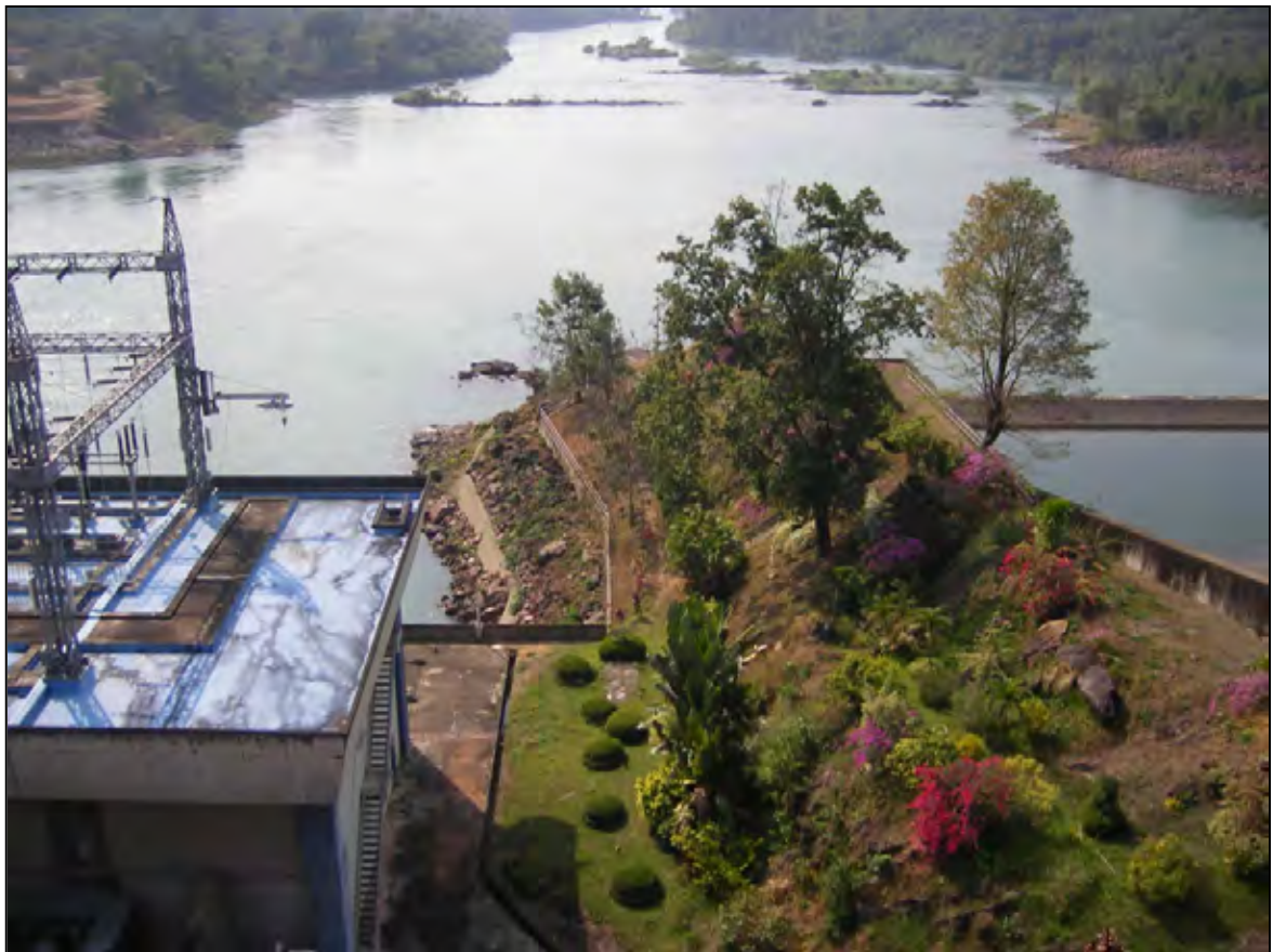
Downstream View from Nam Ngum 1 Dam
