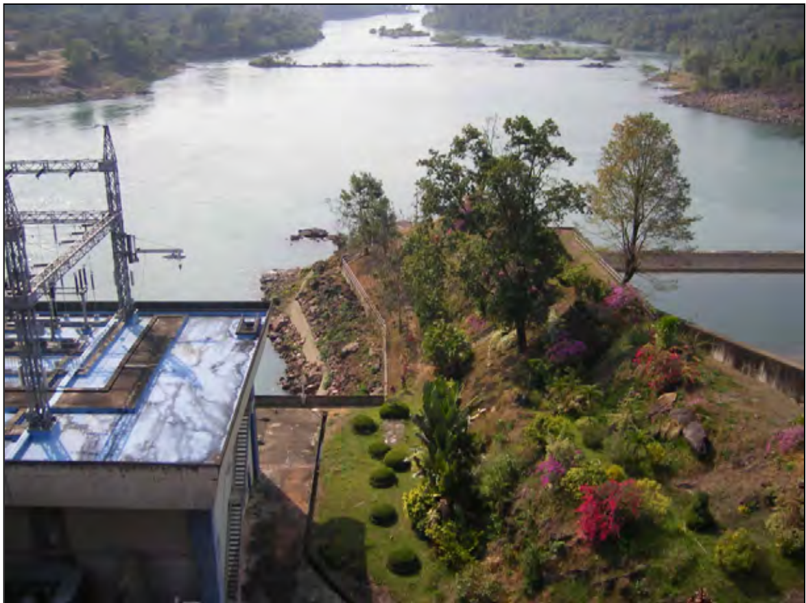
Downstream View from Nam Ngum 1 Dam
