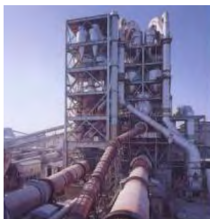
Figure 3.4.8-1 Rotary kiln with NSP.
