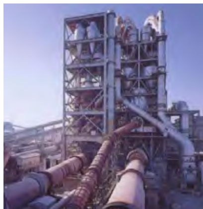
Figure 2.8.5-2 Dry Type Cement Rotary Kiln with NSP
