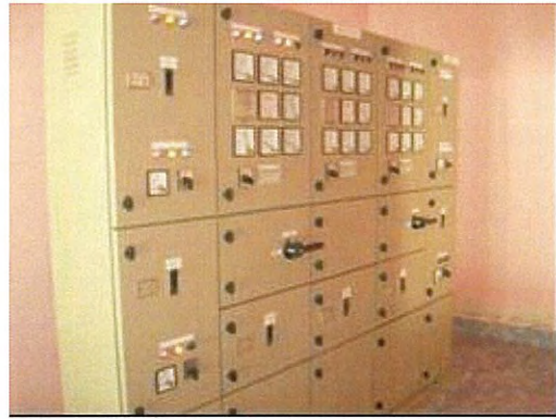
Generator Control and Distribution Panels
