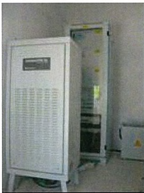
Ex and present inverter
