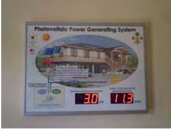
PV generation output display (Island Office)
