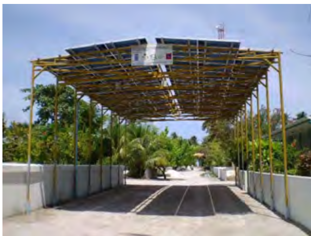
PV panels installed on a roof over an island road
