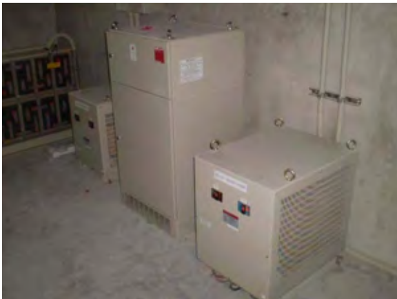
Power conditioners and system transformer (consolidated government offices)
