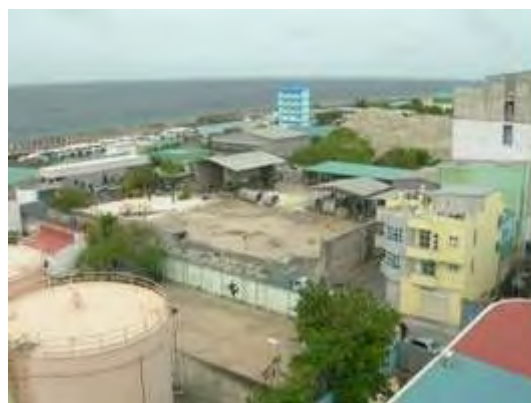
Figure 3.3.4-2 Site for installation of emergency power generating facilities
