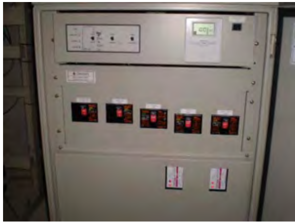
Grid backup board (Island Office)
