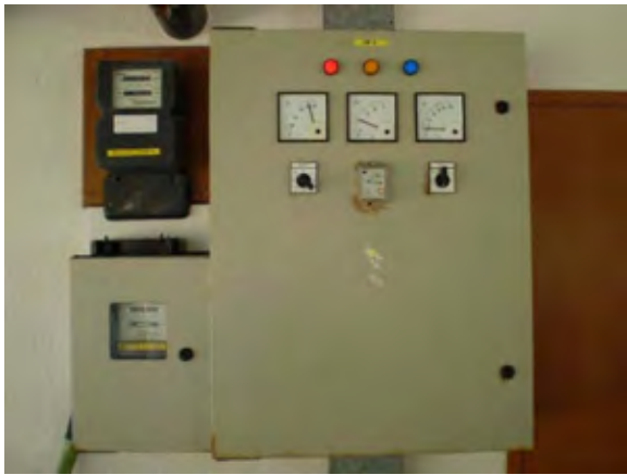
Measuring Unit (top row: excess power measurement; bottom row: consumed power measurement) (Island Office)
