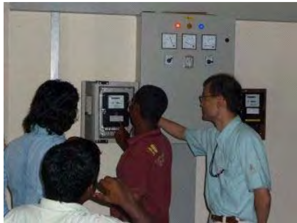
Technical guidance to the MHTE and power plant staff (consolidated government offices)
