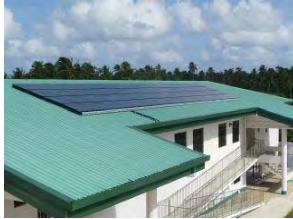
PV array (Island Office)
