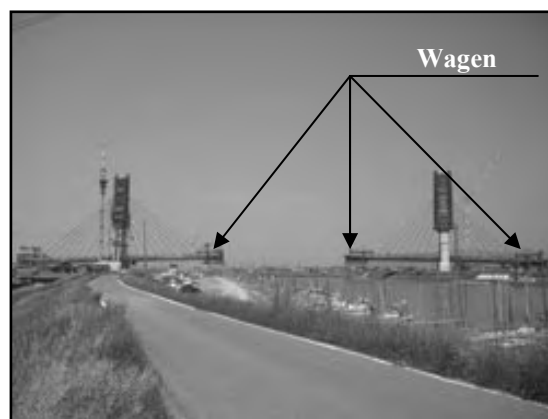
Figure 7.1.7 Construction of PC Girder with Wagens
