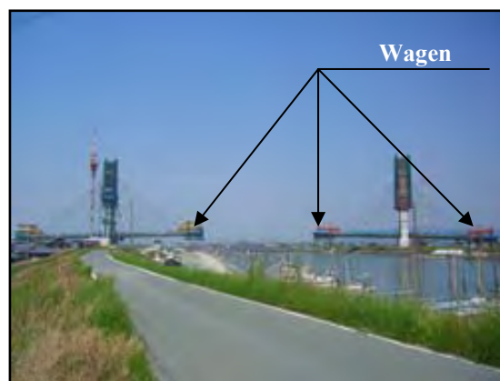
Figure 7.1.7 Construction of PC Girder with Wagens
