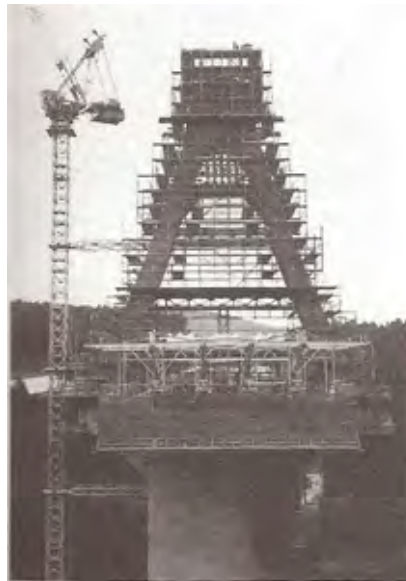
Figure 7.1.6 Construction of Inverted Y-type Pylon with Whole Scaffoldings
