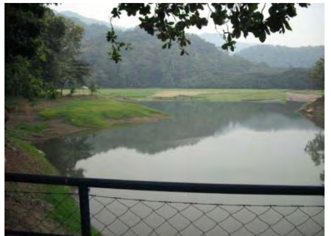
Dam Site for Tisa Water Treatment Plant
