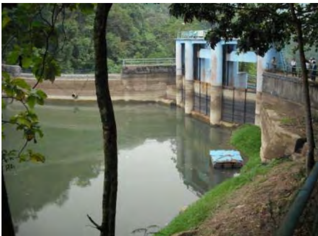
Dam Site for Tisa Water Treatment Plant
