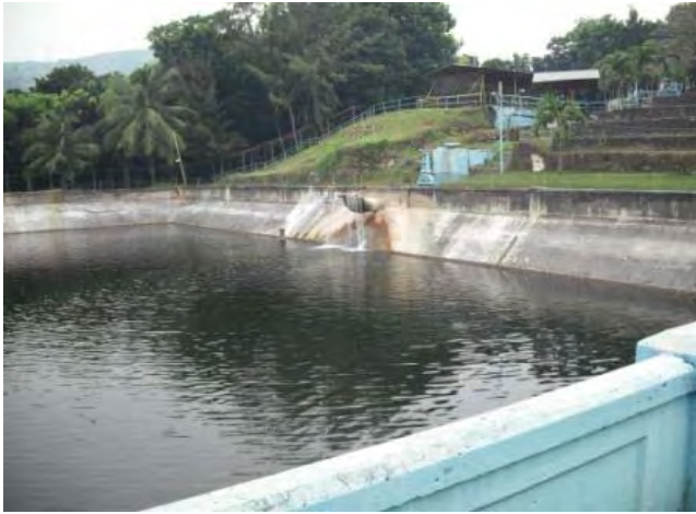
Tisa Water Treatment Plant (1)
