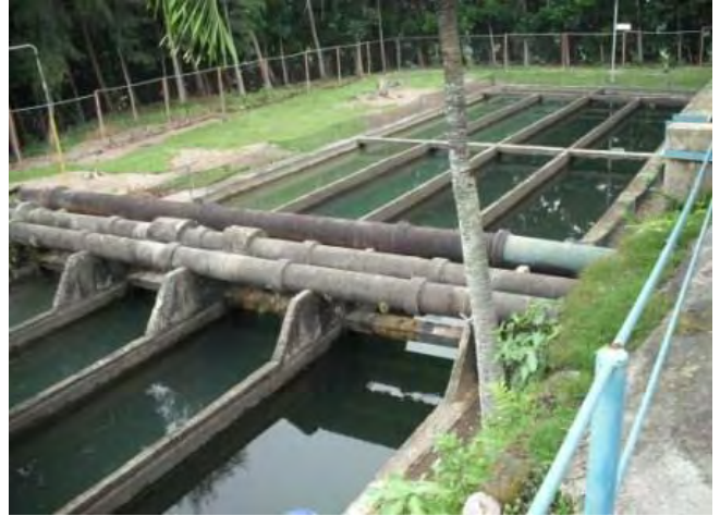
Tisa Water Treatment Plant (2)
