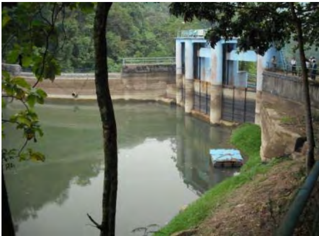
Dam Site for Tisa Water Treatment Plant
