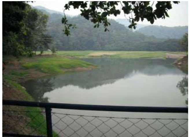
Dam Site for Tisa Water Treatment Plant
