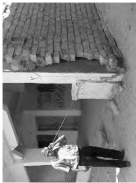
Figure 7-1 Detecting Leakage on House Connection by Acoustic Rod
