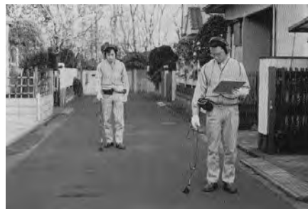
Detection Work by Leak Detector
