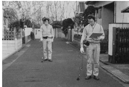
Figure 4.1-11 Work by Leak Detector
