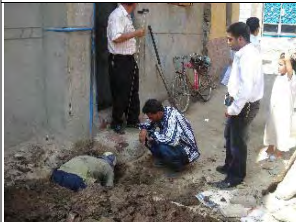
Repairing leakage point in Ibrahimiya. (Action U12). (Date: Jul. 24, 2008)
