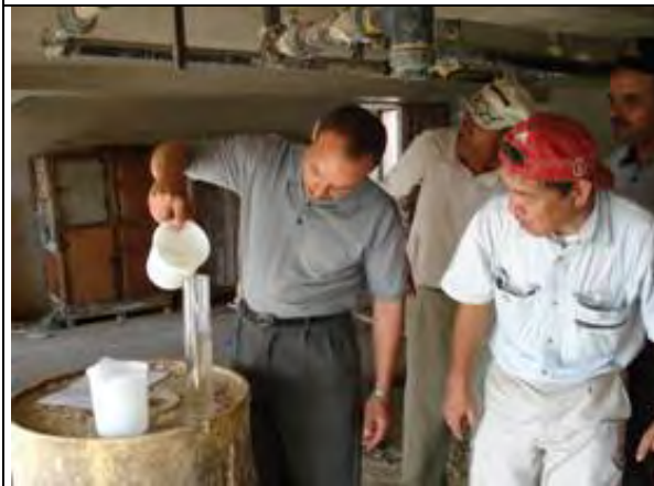
OJT of chlorine control in Abbasa W.T.P (Action S6). (Date: July.17, 2008)
