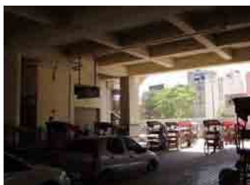
Rickshaws pool under the elevated railway track
