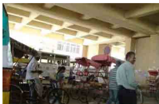
Rickshaws pool under the elevated railway track
