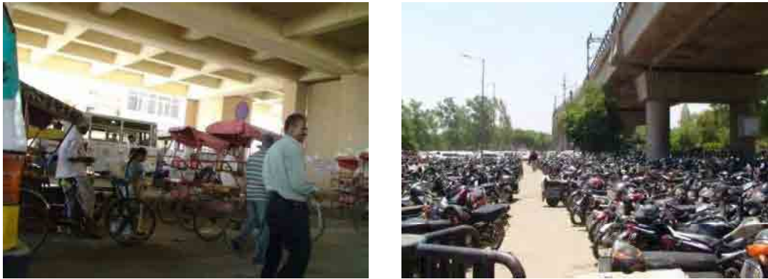
Rickshaws pool and Motorbike Parking under underneath the elevated railway track
