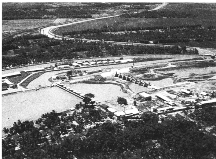
New Lengkong Dam under construction
