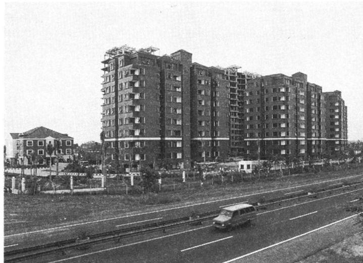
Current photo of downtown Surabaya, marked by high-rise buildings
