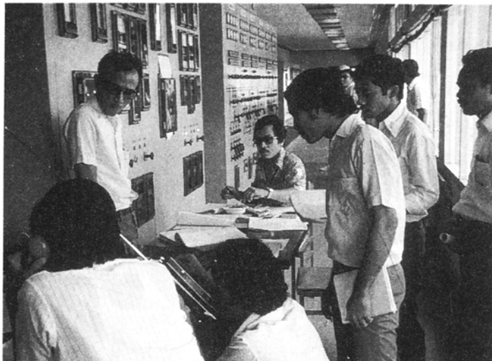
Power transmission test at Waru Substation
