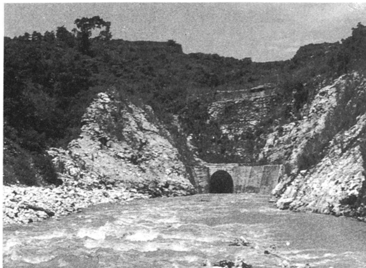
Inlet of Nejama Diversion Tunnel
