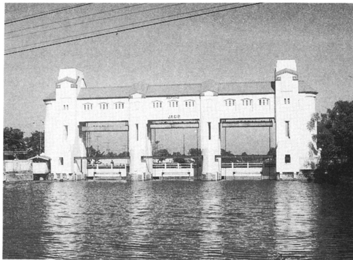
Jagir Water Gate across Wonokromo Discharge Channel
