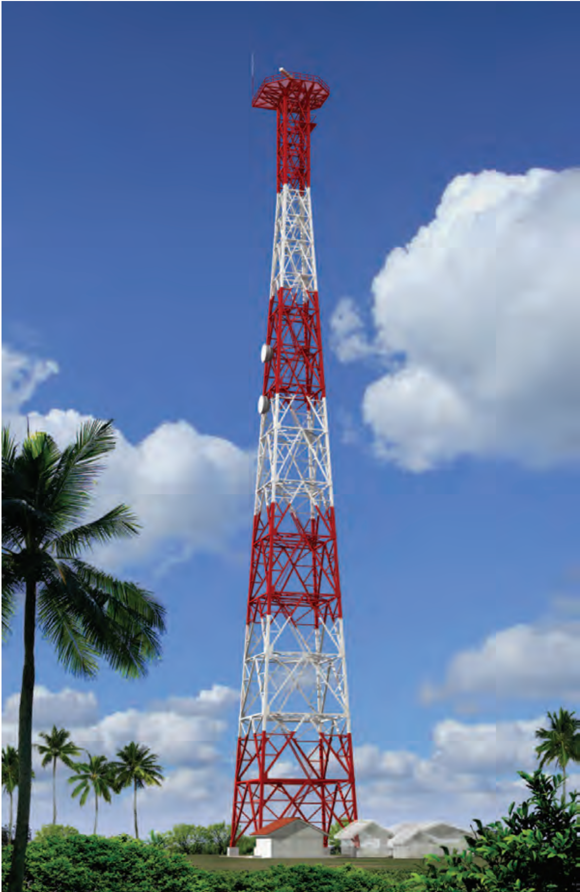
Steel Tower for Radar and Multiplex Communication Links
