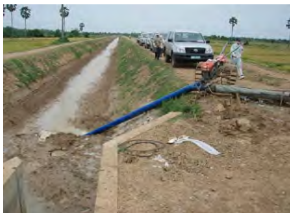
Rehabilitated Secondary Canal (Por Canal Sub-project)
