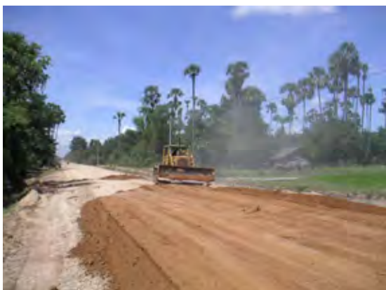
Road under Construction within Command Area (Lum Hach Sub-project)
