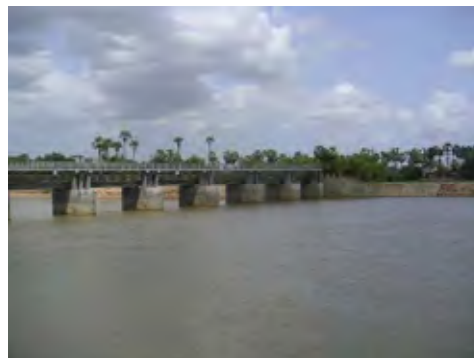
Cha Rec Headworks Completed in 2008 (August 11th, 2009) (Char Rek Weir Construction Project)
