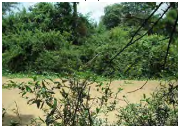
Construction Site for Wat Chre Headworks. (Wat Chre Sub-project)
