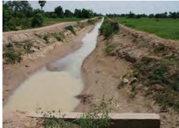
Rehabilitated Secondary Canal (Damnak Ampil Sub-project)
