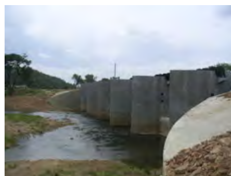
Spillway Completed in 2009 (August 10 th , 2009) (Bassac Reservoir Rehabilitation Project)
