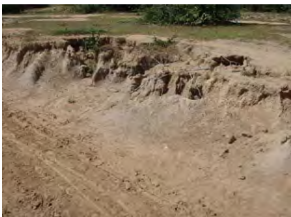
Present Condition of Main Canal (Wat Loung Sub-project)
