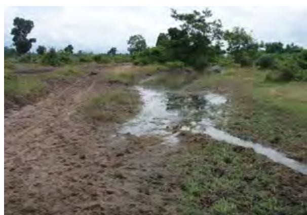
Present Condition of Main Canal (Lum Hach Sub-project)
