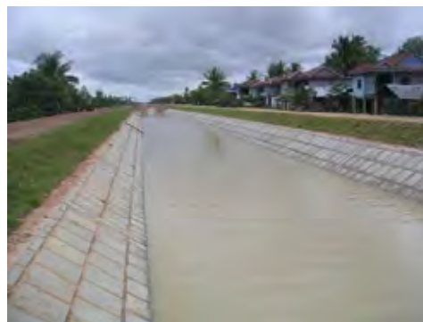
Main Canal Rehabilitated (July 11 th , 2007) (Kandal Stung Irrigation Development Project)
