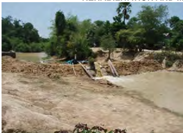
Present Condition of Secondary Canal (Wat Chre Sub-project)
