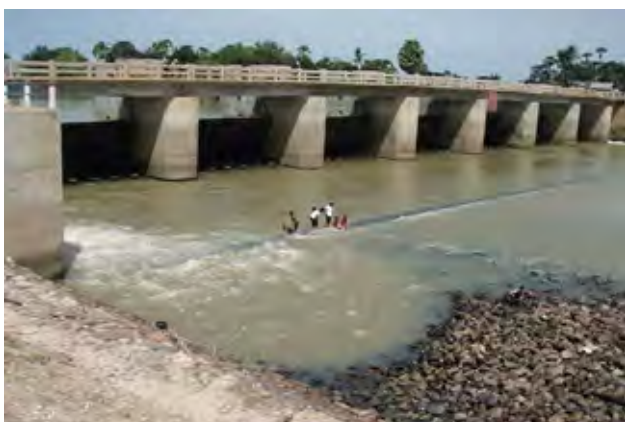
Existing Damanak Ampil Headworks (Damnak Ampil Sub-project)
