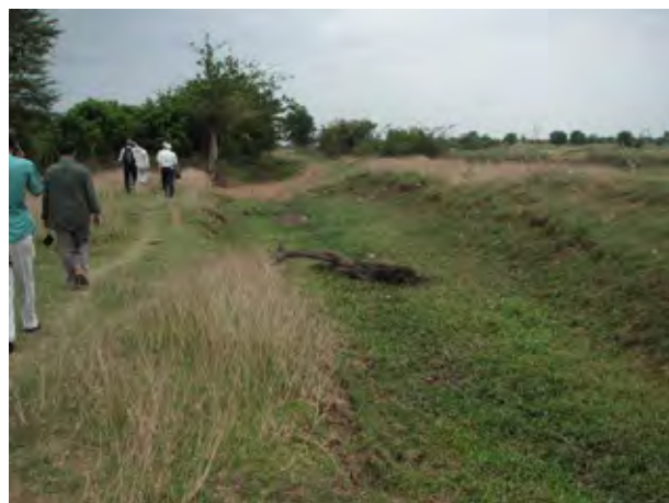
Present Condition of Main Canal (Ream Kon Sub-project)
