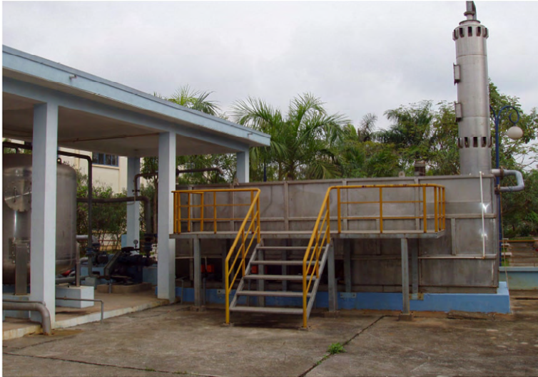
College of Urban Works Construction
