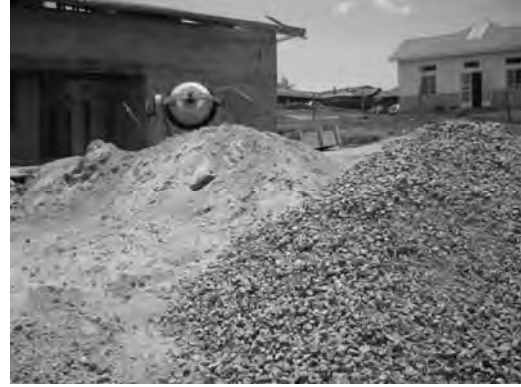
Photo: Field Concrete Mixing, Aggregate Stockyard
