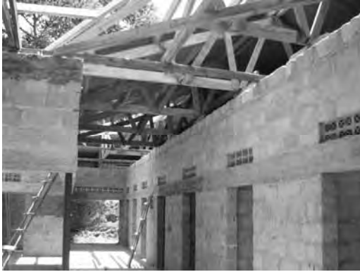
Photo: On going Construction Site, Masaka RRH
