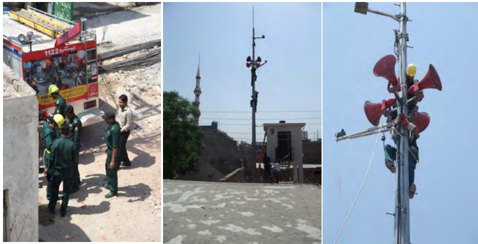
Fig. 4-3 Repairing Work of Speaker Cable at Warning Post WP-2
