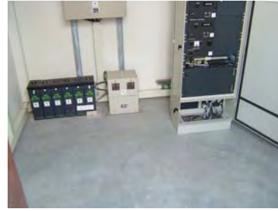
Warning Post (after)
